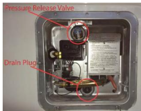
Figure 4 Pressure Release Valve and Drain Plug Locations
