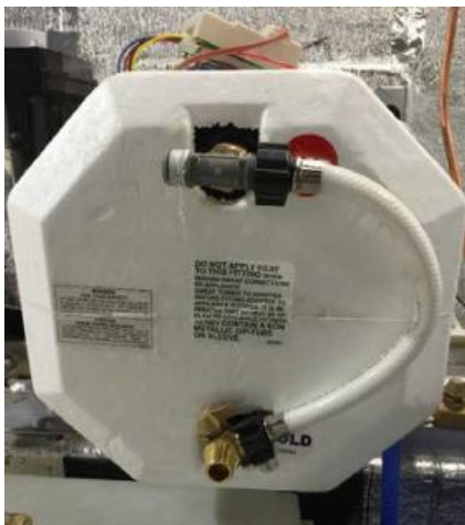
Figure 1 Water Heater Bypass Assembly
