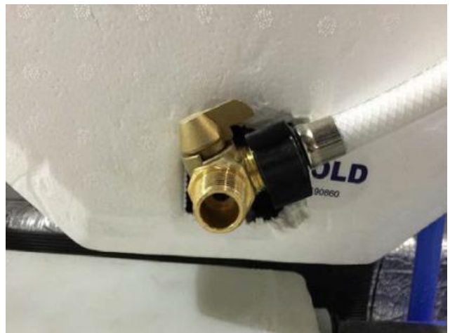
Figure 2 Water Heater Valve in Bypass Position
