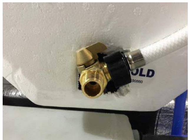
Figure 2 Water Heater Valve in Bypass Position
