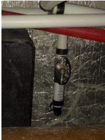
Figure 3 Valve in Open Position
