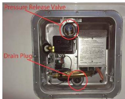
Figure 4 Pressure Release Valve and Drain Plug Locations
