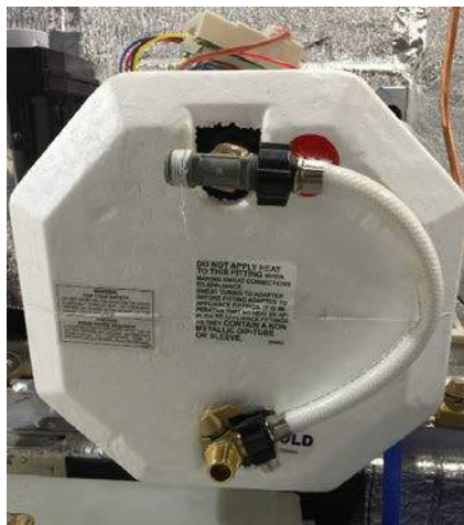
Figure 1 Water Heater Bypass Assembly
