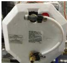
Figure 1 Water Heater Bypass Assembly
