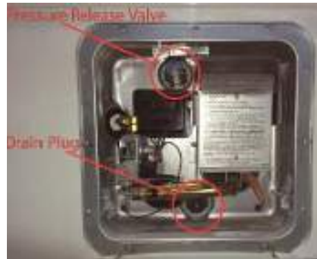
Figure 4 Pressure Release Valve and Drain Plug Locations
