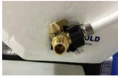
Figure 2 Water Heater Valve in Bypass Position
