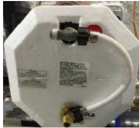
Figure 1 Water Heater Bypass Assembly
