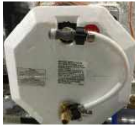
Figure 1 Water Heater Bypass Assembly
