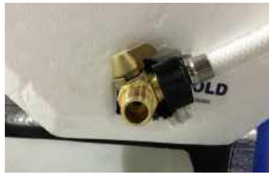
Figure 2 Water Heater Valve in Bypass Position
