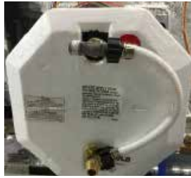
Figure 1 Water Heater Bypass Assembly
