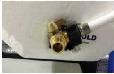
Figure 2 Water Heater Valve in Bypass Position
